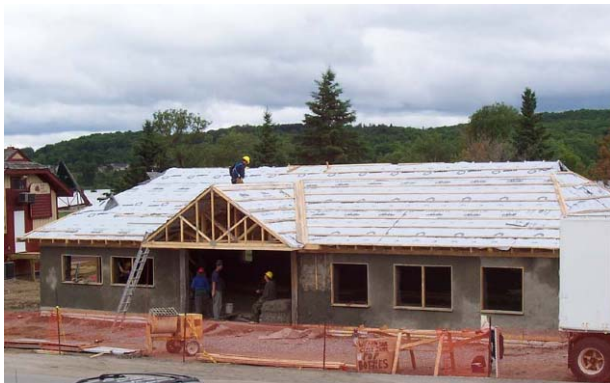
the walls after plaster has been applied.
